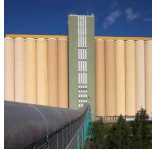
Reparations of grain infrastructure, Köping
